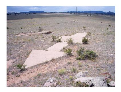
These old planes couldn't rely on radio much of the time, so they used these arrows, along with beacon towers, to navigate.
